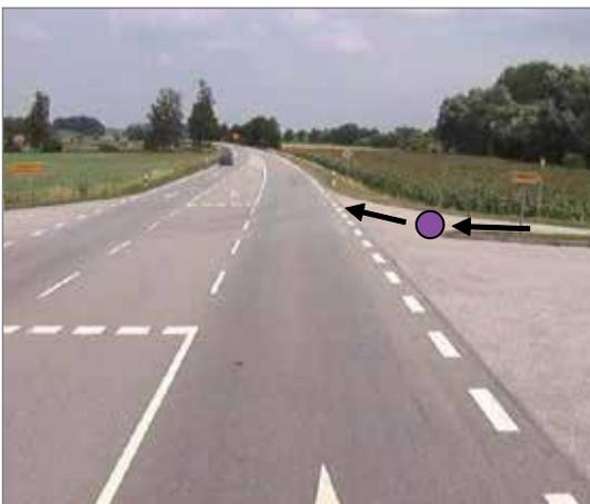
The large waiting area on the minor road incited drivers to enter the major road too quickly, which caused conflicts when decelerating and resulted in rear-end collisions.
