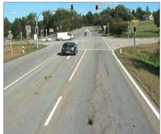
A separate left-turn phase “protects” road users turning left into the minor road from encountering oncoming traffic.
