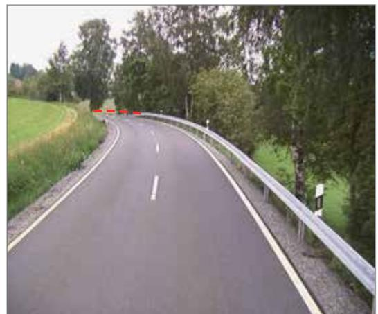
Passive safety was increased by means of a steel crash barrier.
