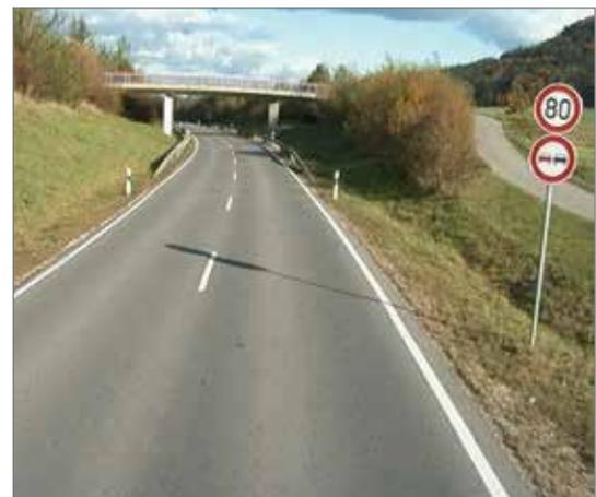
The ban on overtaking prohibits overtaking in the area of the bend. The speed limit reduces the speed level.
