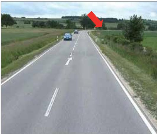
The intersection was hard to see. Drivers overtook other vehicles before the intersection, which caused them to recognize vehicles turning too late and the following traffic collided with the vehicle's rear end.
