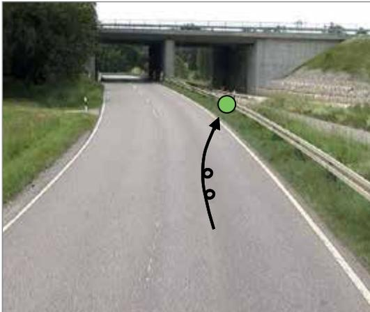
The centre road marking was in a poor condition and could hardly be seen at all. In addition, it was hard to see the further direction of the road due to a bridge, which promoted single-vehicle accidents.
