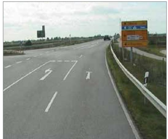
The remodelling of the intersection according to the regulations including a modified right of way creates an unambiguous right of way situation.
