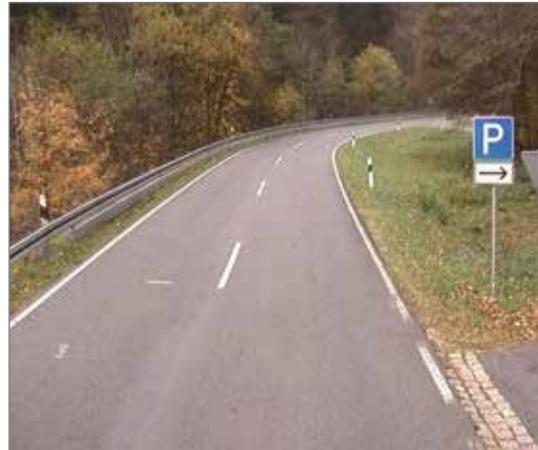
Passive safety for motorcycle riders was increased by means of an underrun protection. **BUT:** The edge marking is still in need of improvement.
