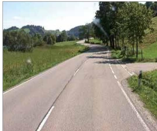
Visibility was improved by removing the obstacle (tree).
