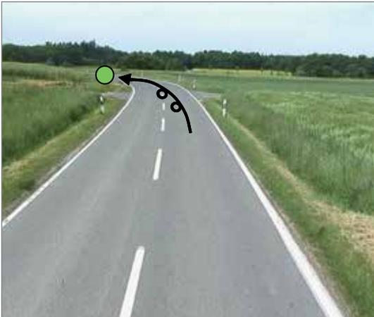
The layout of the road was discontinuous and the double bend could not be seen, which promoted single-vehicle accidents.
