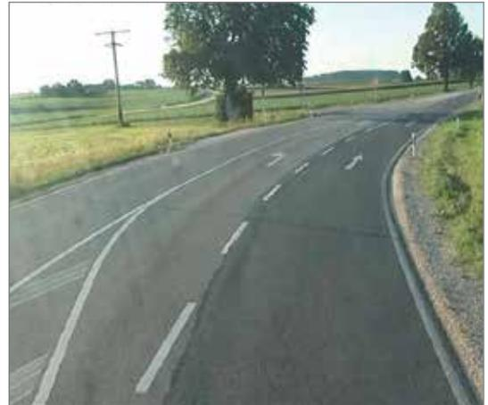
The added left-turn lane improves the visibility of the intersection on the major road and enables left turns without any danger to following straight-through traffic.
