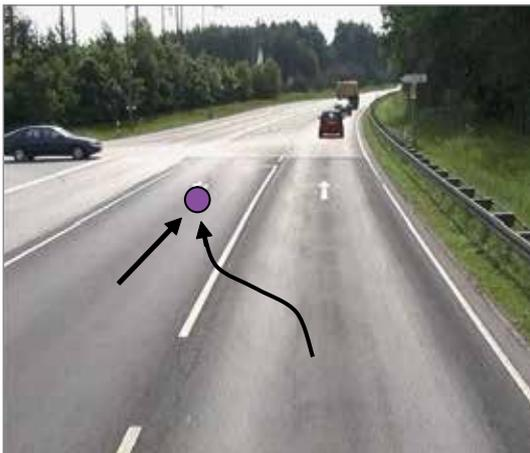
High driving speeds and high traffic volumes on the major road incited drivers to initiate risky lane changes ahead of the intersection which caused rear-end collisions with following vehicles.
