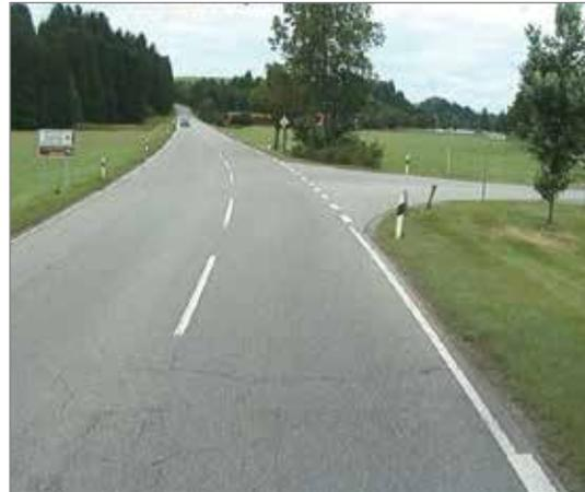
Obstructions reducing visibility for traffic turning into the major road were removed by optimising the installation sites of the signs.
