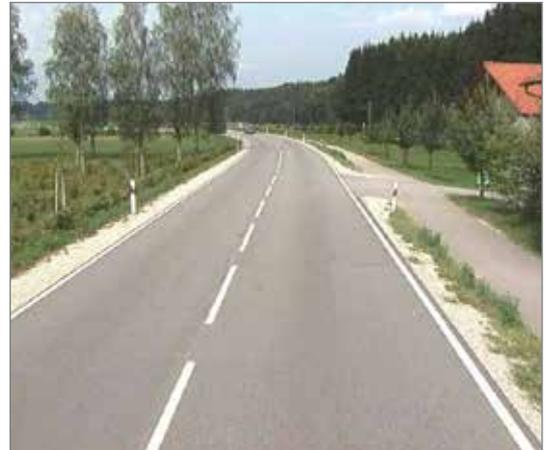
Thanks to the extension work based on the existing structure, the road is safe for traffic again. **BUT:** The vegetation in the inner bend is still limiting visibility. In addition, the safety distance between the road and the attached bicycle path is insufficient.
