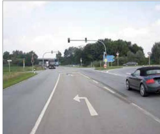
A traffic light system provides sufficiently long time gaps in the main flow for safe turning into/crossing of the major road. In addition, the separate left-turn phase provides increased safety when turning.
