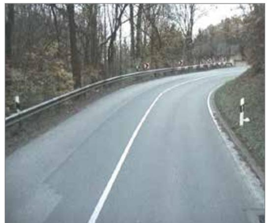
Individually placed bend chevrons indicate the direction of the bend on an extended stretch of road. **BUT:** Visibility is still limited by the slope in the inner bend.
