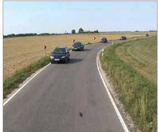
Individually placed bend chevrons and renewed road edge markings indicate the direction of the bend.
