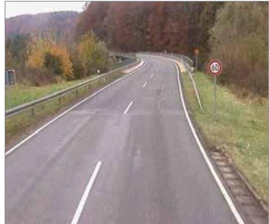
The speed limit reduces the speed level before the critical section of the road. In addition, the road surface beyond the accident blackspot was repaired.
